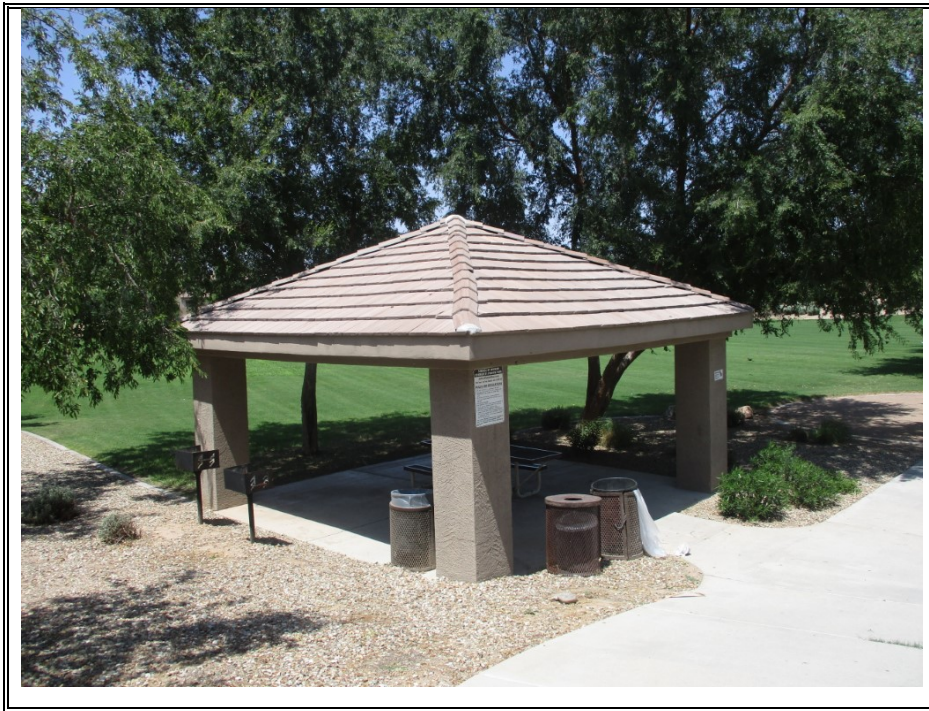
CONCRETE TILE ROOF (TYPICAL)
