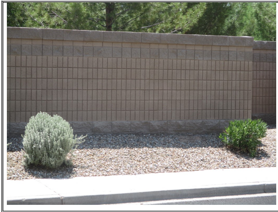
CONCRETE BLOCK WALLS (TYPICAL)
